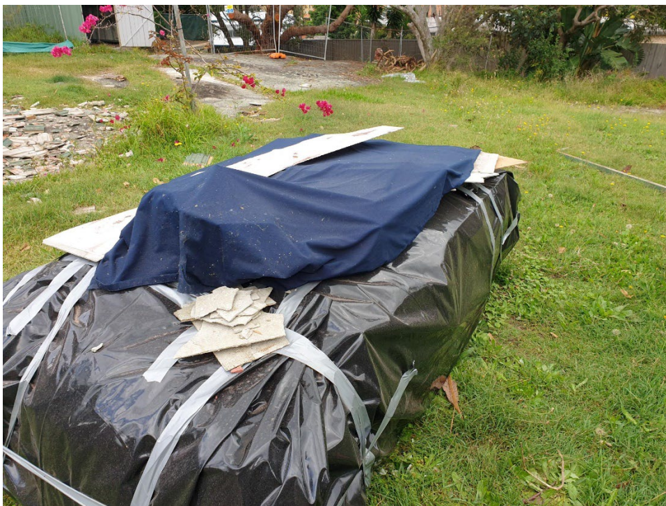
Photo 3: Example of asbestos waste “parcel” not suitably sealed, contained and secured in a manner that facilitates its future safe disposal, with apparent additional unwrapped asbestos-containing material added.
